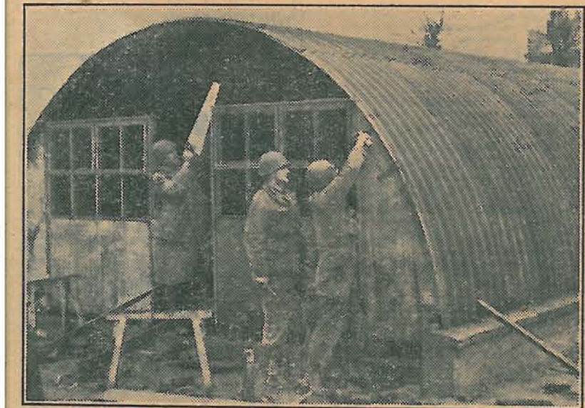
U.S. engineers repairing bomb-damaged homes in London's Lambeth area cleared this blitzed site and erected a temporary house in seven days.
